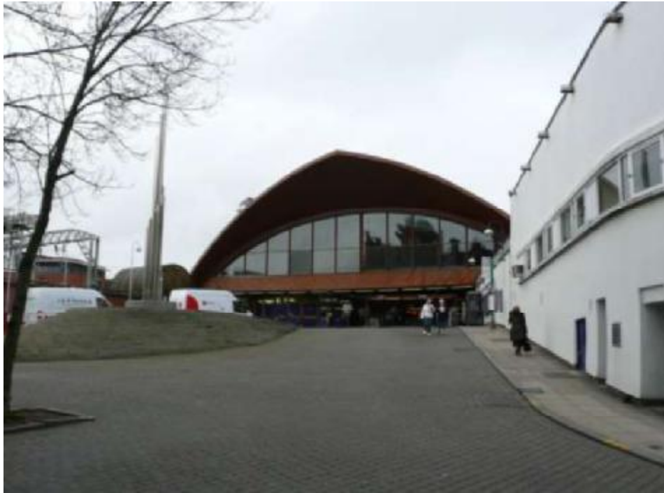
Oxford Road Station
